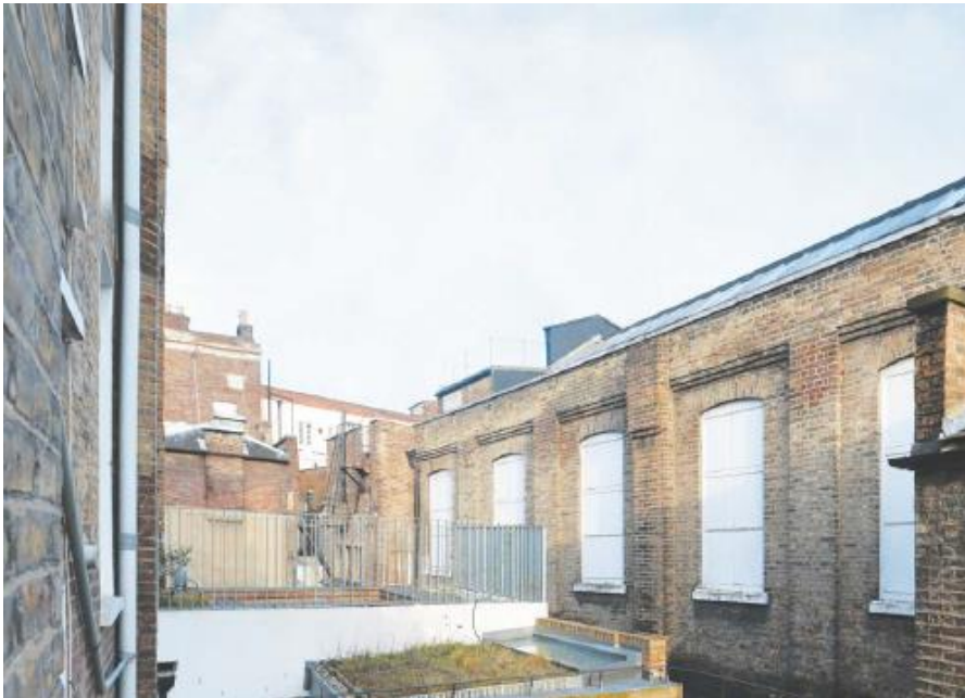
Photograph 6: Looking towards the terrace at 84 Queens Head Street and the windows of 162 Packington Street
